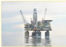
Petroleum and chemical industry
